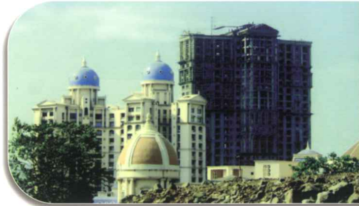
Pozzocrete™ at work Hiranandani project, Mumbai
