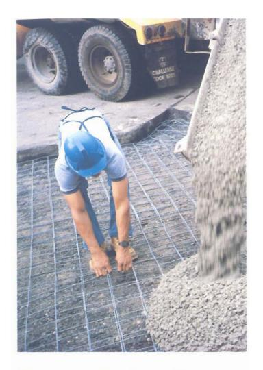
Today, you do not have to settle for the wire mesh method and gamble on it being in the right place. With the Fibermesh® family of fibres, an alternate reinforcement system, the formation of cracking during the plastic stage of concrete is reduced. It also eliminates the hassles associated with welded wire fabric (WWF).
